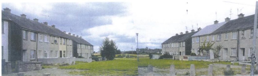
VIEW OF LINK BETWEEN CARBURY PARK & TOWNSPARK
